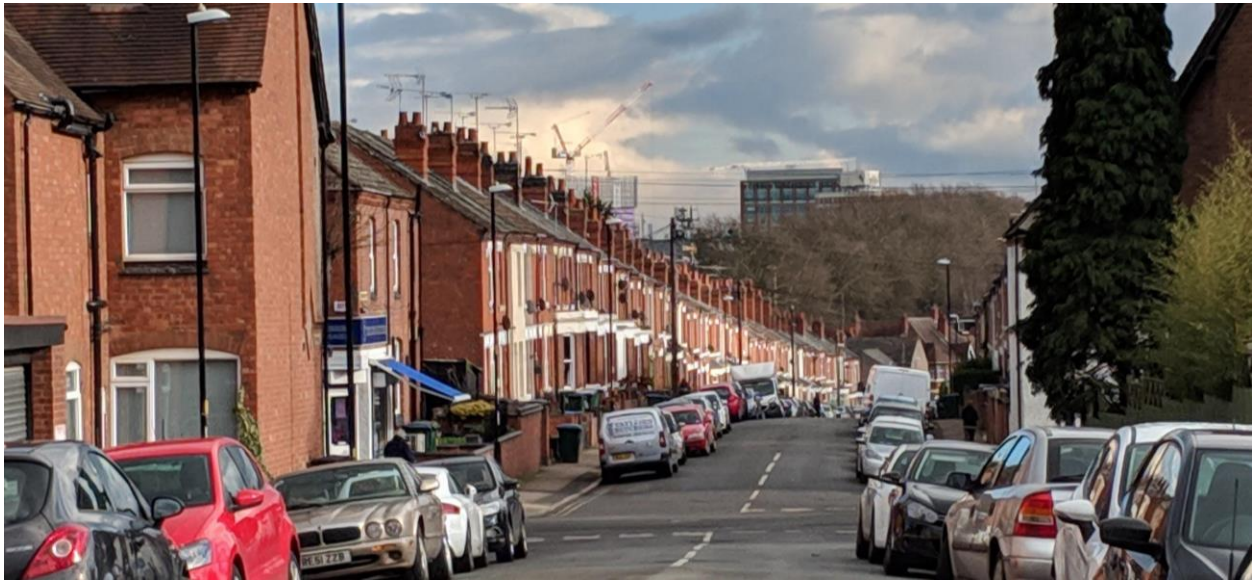
Fig 3.19. Newcombe Road provides views back to the City Centre. Despite a strong terrace rhythm with a run of smaller-scale red brick terraces incorporating chimneys and stone detailing enhanced by a curving street structure, the group has been undermined by visual clutter including satellite dishes, tv aerials, bins, as well as alterations to windows and front boundary treatments.
