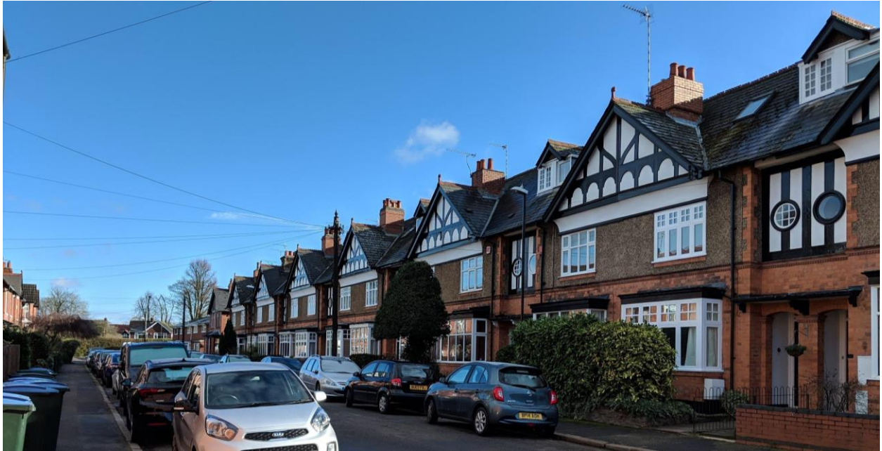
Fig 3.14. To the east side (right) of Avondale Road there is a terrace with a highly significant surviving decorative pattern incorporating half-timbered gables topped with roof finials, chimneys, bay windows, a contrast between brick and roughcast render (separated by brick banding) and round oculi windows. Whilst the terrace is enhanced by front boundary soft landscaping, there has been loss of historic boundary treatments and hard-standing/surface materials.
