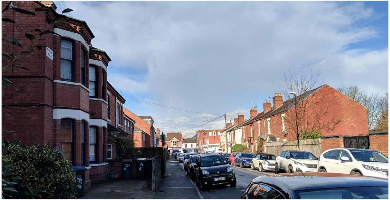
Fig 3.8. Providence Street provides important views down to Earlsdon St with a series of smaller-scale red brick terraces which are unfortunately impacted by infill and visual clutter to facades, including satellite dishes.
