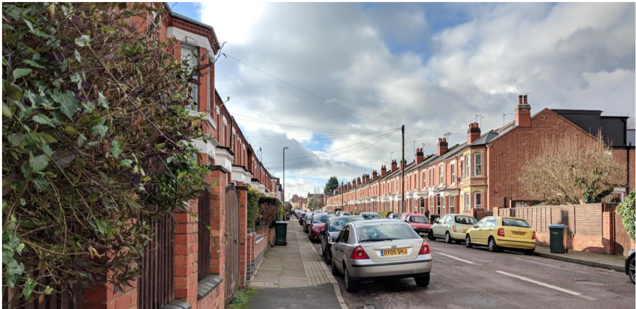
Fig 3.27. Berkeley Road North is characterised by significant groups of red brick terraces (with some examples of roughcast render) incorporating stone banding and hoods around windows and doors some of which incorporate a pattern, as well as key features such as chimneys which provide a strong rhythm to the road. Despite a strong terrace rhythm many historic windows have been lost, boundaries rebuilt and at least one example of a red brick facade being inappropriately rendered.
