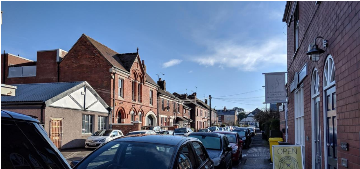
Fig 3.6. Moor Street incorporates a former nail factory, now converted to offices, alongside a series of terraces with some later infill. Key losses along this road include historic boundary treatments (rebuilt), and windows. At least one brick terrace has been inappropriately rendered. The Criterion Theatre, provides an important visual terminus to the road.
