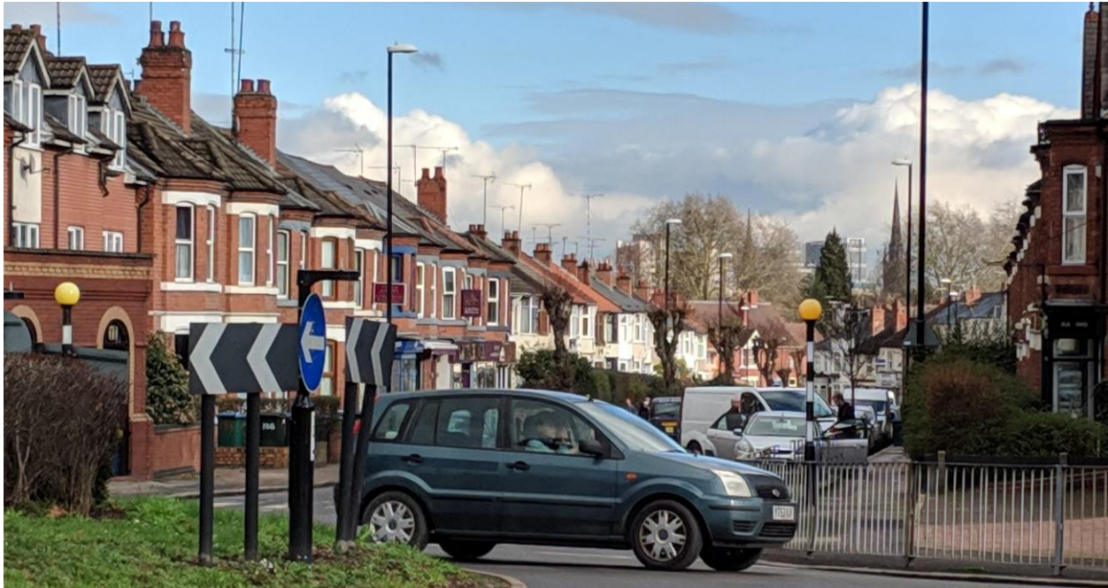
Fig 3.18. The junction allows significant views back to the City Centre, including those of Coventry's medieval spires.
