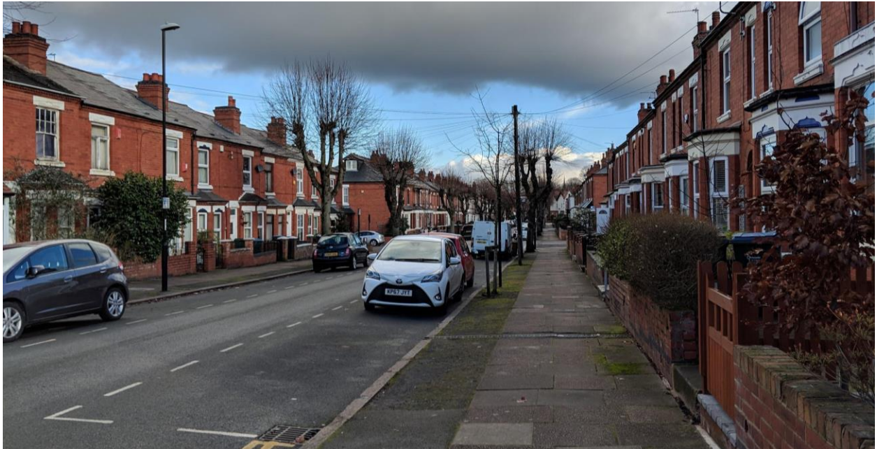
traditional sash windows remain, many have been replaced with uPVC top hung windows and traditional boundary treatments have been rebuilt.
